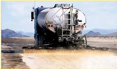
Traffic on a ROAD OYL® surface will compact the road into a smooth dust free pavement-like surface.
