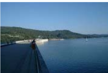
A power plant in Poland
