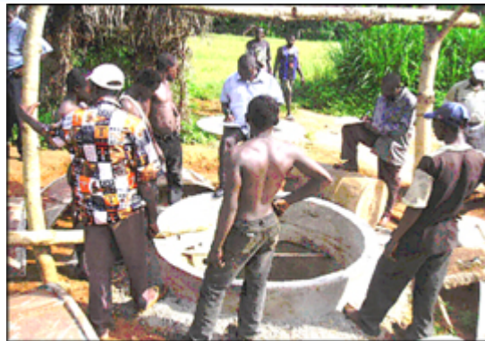
Community work in progress. Water well at Kassana Community Health.
