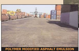
**Polymer modification** changes the flow properties of the liquid asphalt so it can stand up to the sun, wind, weather and traffic loadings.
