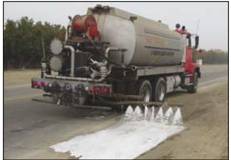
Soil-Sement® being applied.
